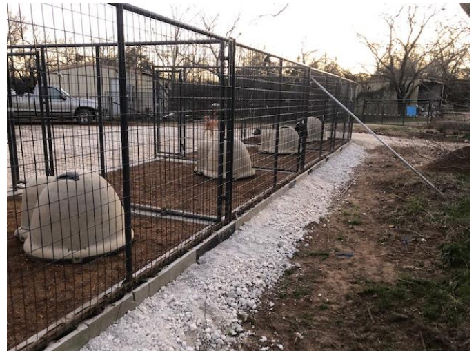
Pens are installed and secured to cement blocks. This cement will prevent rusting of the bottom bars.
