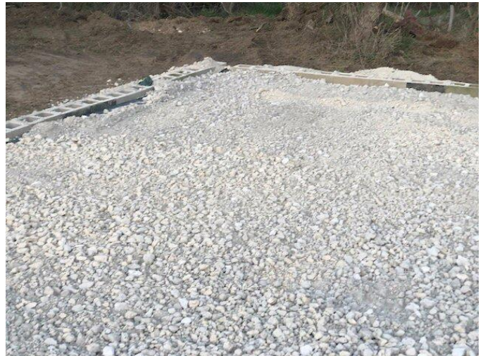
Drains are placed, area leveled and road base applied.
